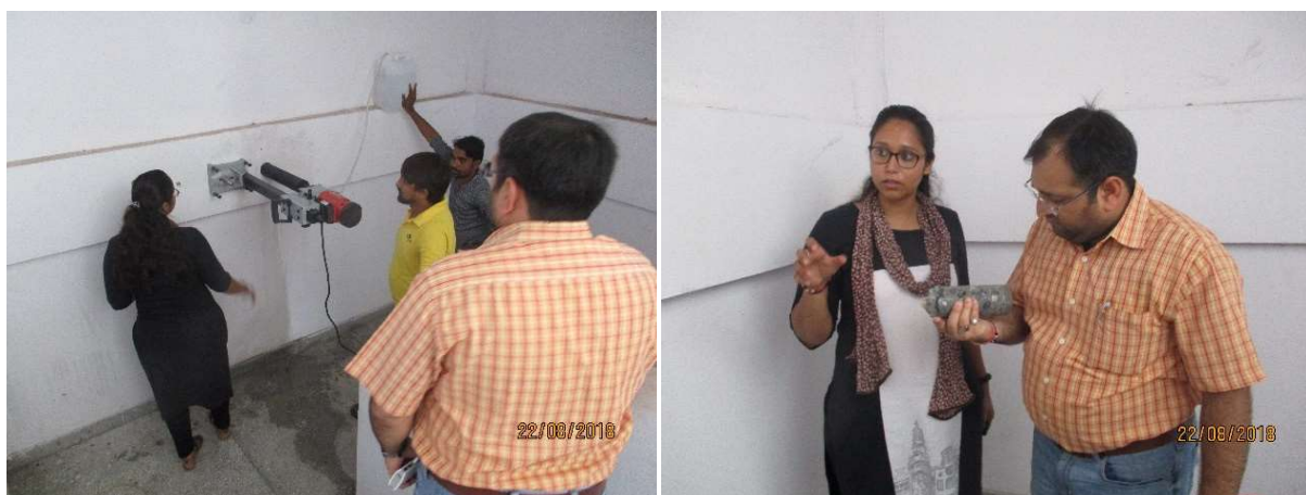
Figure B.9: Core Samples being collected for testing in laboratory
