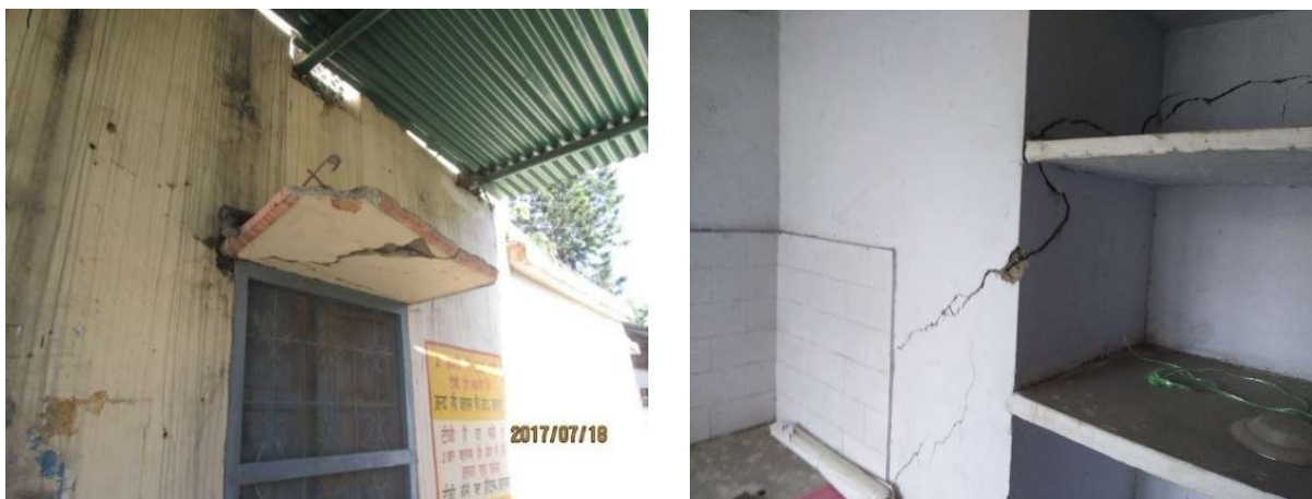
Figure B.3: Structural Distress observed during Visual Survey
