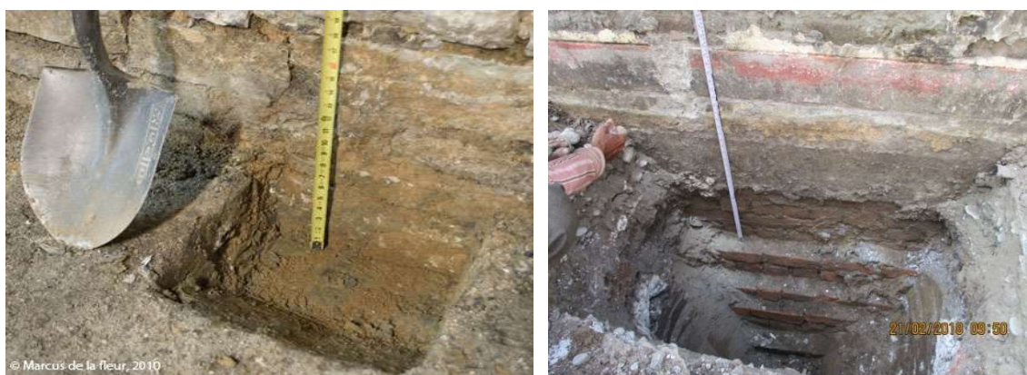
Figure B.6: Trial Pits excavated to expose footing for taking measurement and testing
