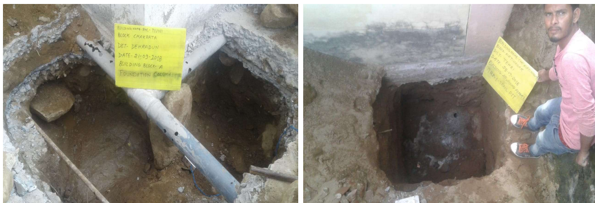
Figure B.11: Trial Pits at Base of Corner Columns
