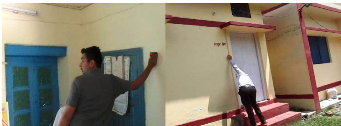
Figure B.2: Measurement being carried out on site for preparing As-Built Drawings
