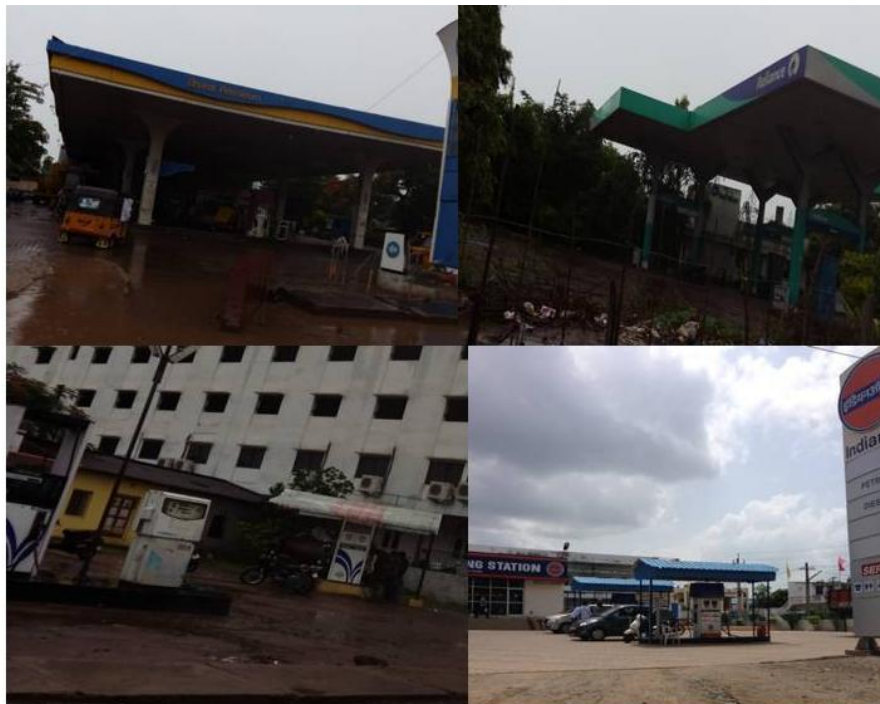
Figure 8-10: Sample photographs of petrol pumps
