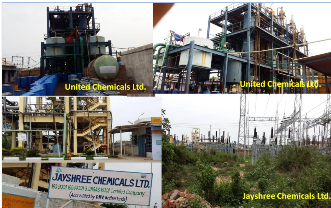
Figure 5-11: A snap shot of industrial buildings in Ganjam district
