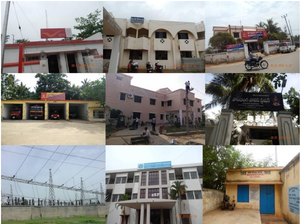
Figure 8-7: Sample photographs of other type of buildings
