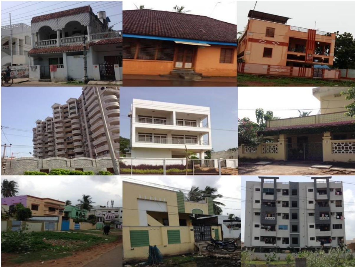
Figure 8-2: Residential buildings in urban areas
