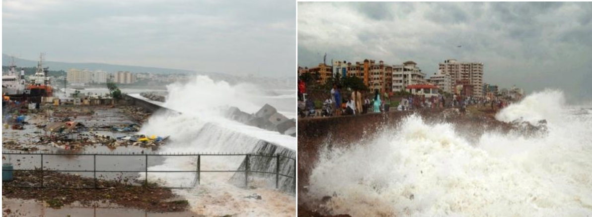
Figure 5-2: Few Damage Photographs associated with Very Severe Cyclonic Storm Phailin ( https://www.google.co.in/ )
